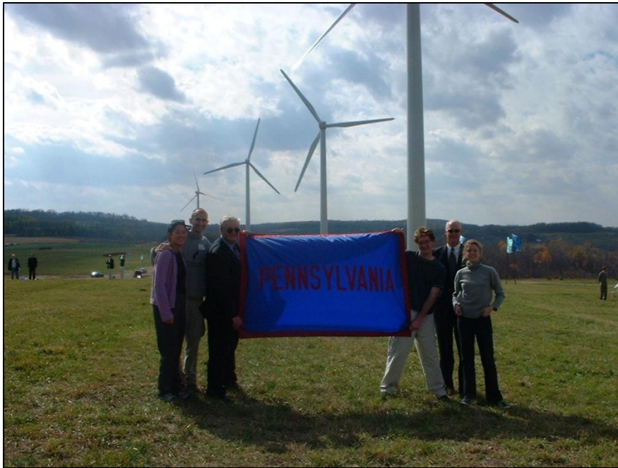
Somerset Wind Farm, PA
