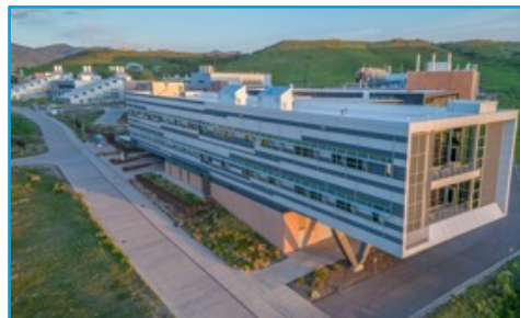
Energy Systems Integration Facility
