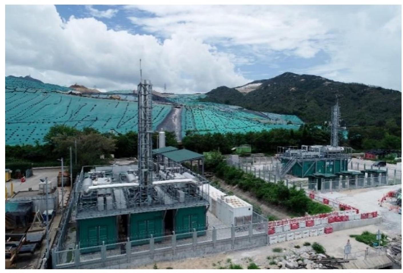
The WE Station at the West New Territories (WENT) Landfill at Nim Wan in Tuen Mun – Hong Kong's largest facility using landfill gas for electricity generation installed by CLP Power and to which the AirTrunk solution will be linked.
