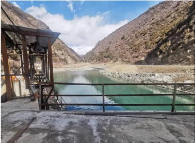
Figure 8 Jiema river at the dam of Jiema station (upstream)
