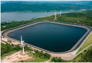
Lamtakong Power Plant
